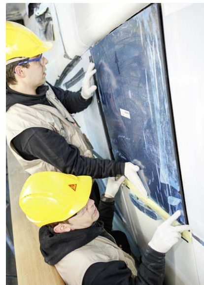
Fig. 7 The window is fitted
